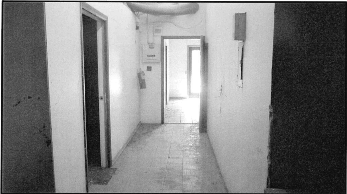
PHOTOGRAPH NO. 2 Looking south (first floor).
