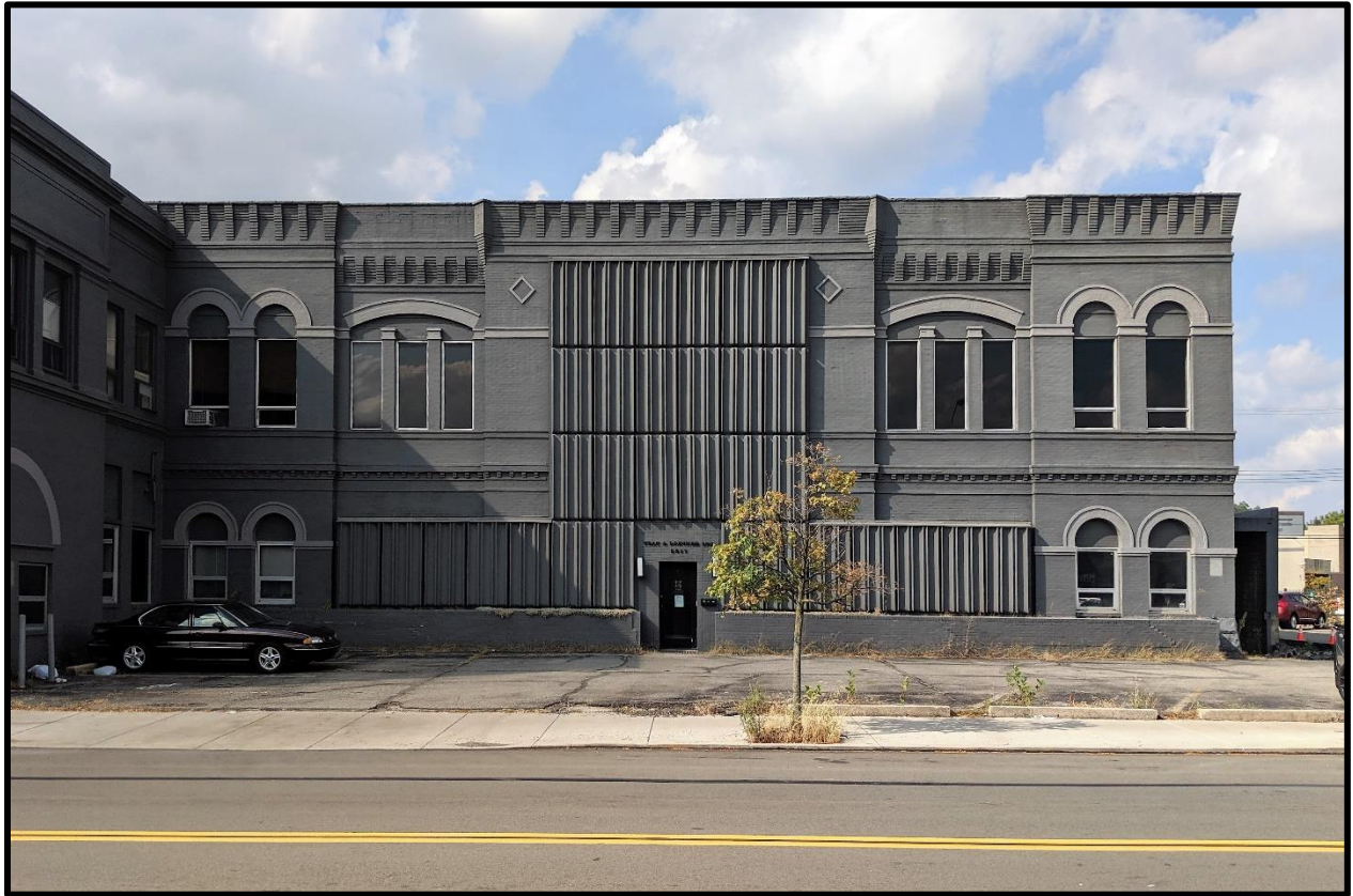
Photo 2: Detail, southeast (primary) façade of 1906 building from Centre Avenue, facing northwest.
