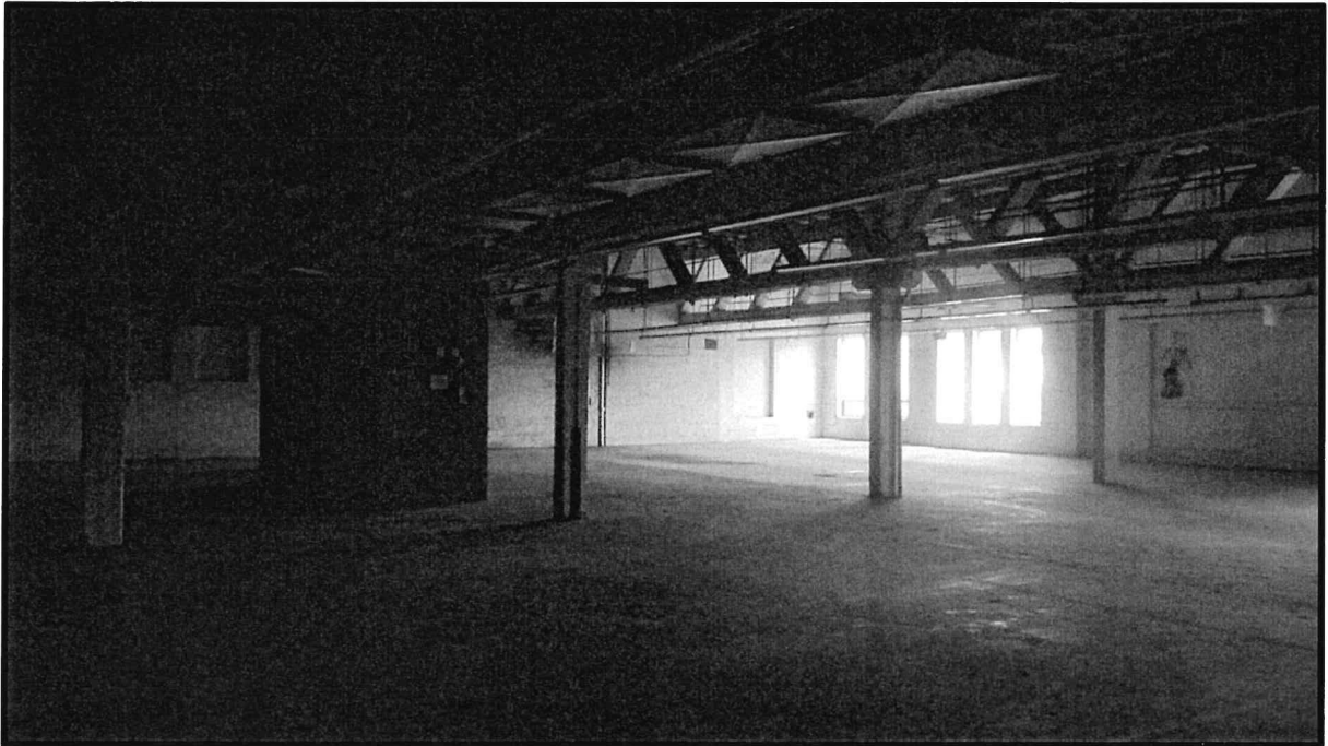
PHOTOGRAPH NO. 5 Looking south (second floor).
