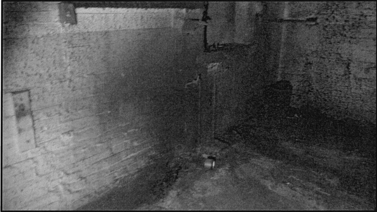
PHOTOGRAPH NO. 9 Looking northeast (second floor).
