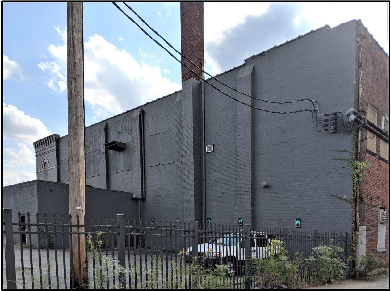
Photo 6: Detail, northeast (side) façade of 1906 building from Commerce Way, facing southwest.
