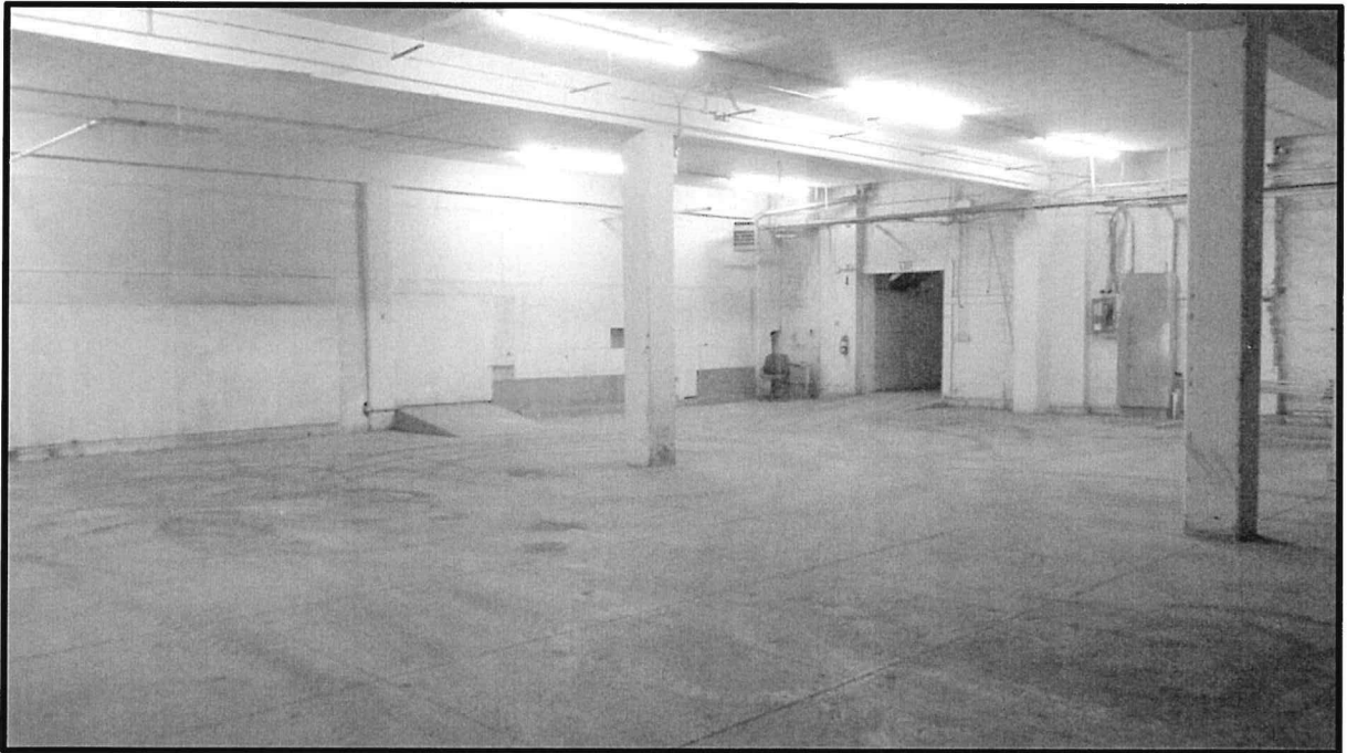
PHOTOGRAPH NO. 4 Looking northeast (first floor).
