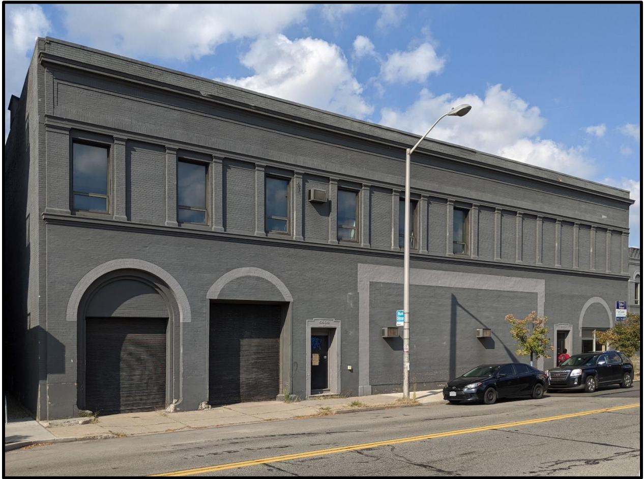
Photo 4: Detail, southeast (primary) façade of 1926 addition, facing northeast.
