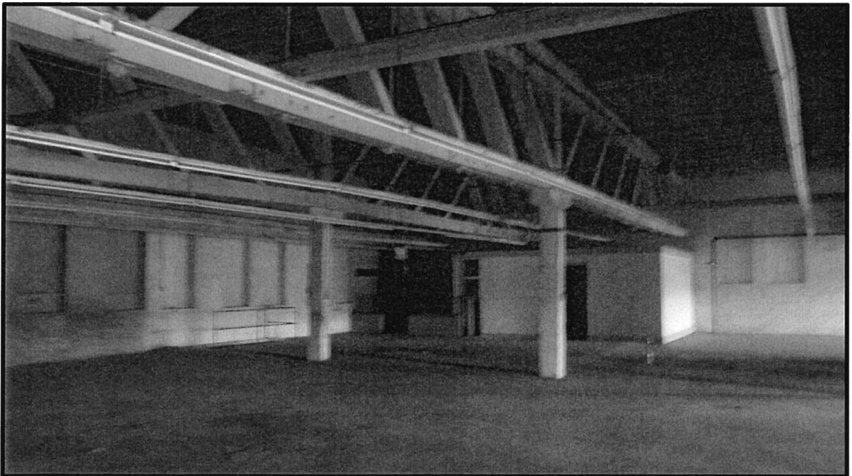
PHOTOGRAPH NO. 6 Looking northeast (second floor).
