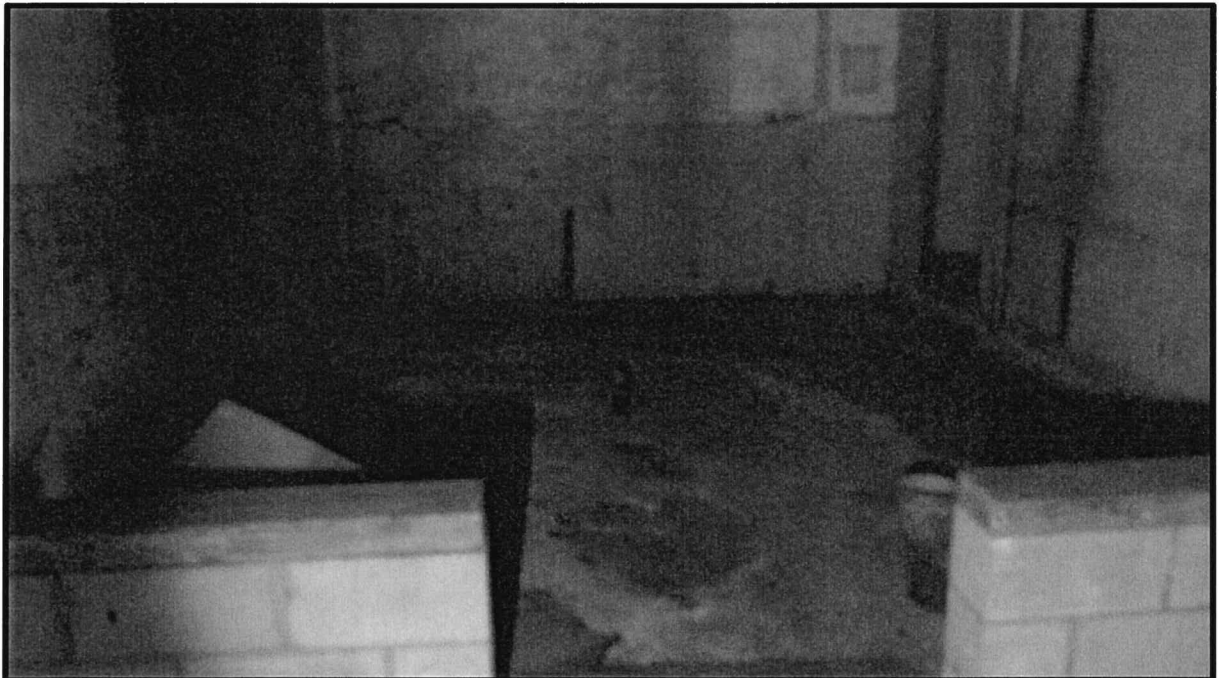
PHOTOGRAPH NO. 8 Looking south (second floor).
