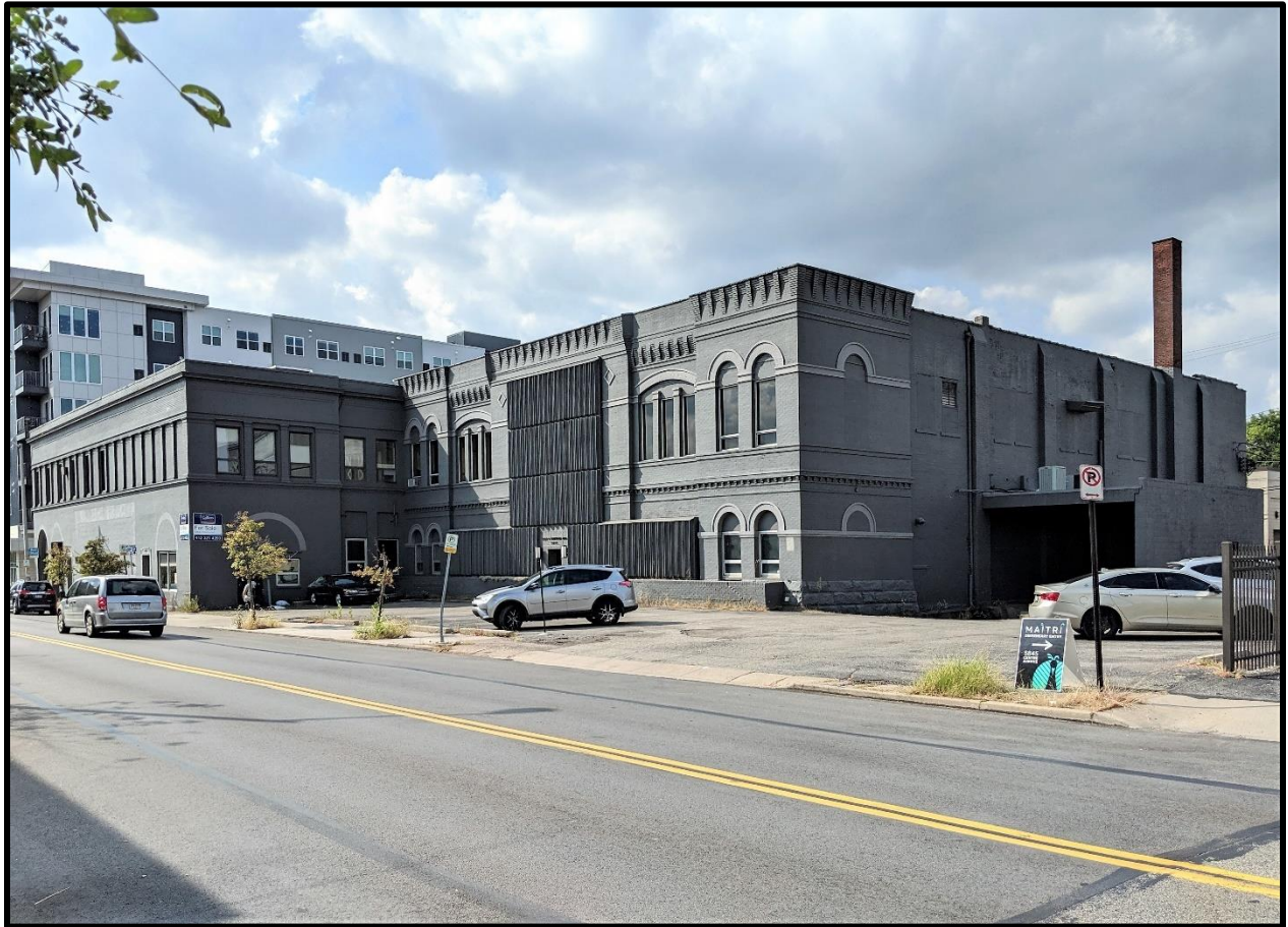
Photo 1: Overview, Hiland Automobile Company Building, southeast (primary) façade and northeast (side) façade, facing northwest from Centre Avenue. 1906 building (set-back from Centre Avenue) visible at center-right. 1926 addition (built to lot line) visible at left.
