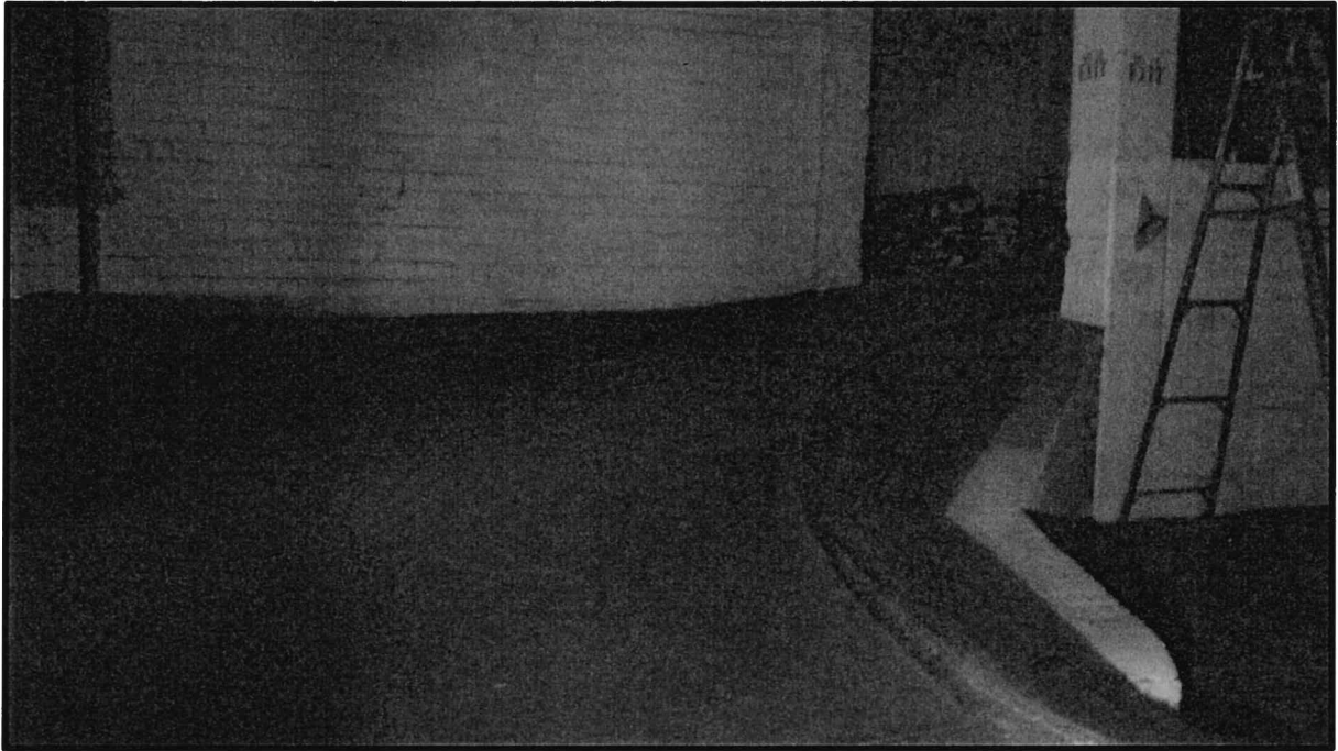
PHOTOGRAPH NO. 7 Ramp to roof looking northwest.
