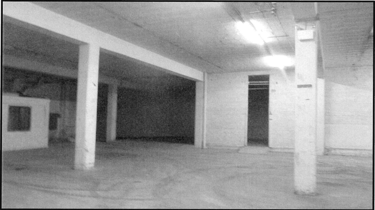
PHOTOGRAPH NO. 3 Looking southwest (first floor).
